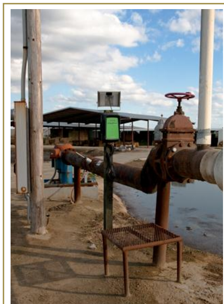
Affordable flow meters for measuring dairy lagoon water are available with solar or battery power, data loggers and wireless data transfer. The right flow meter can greatly simplify nutrient management recordkeeping, and, when installed with a throttling valve or variable frequency drive controller, make it possible to accurately apply the specific amounts of nitrogen called for in the nutrient plan.
