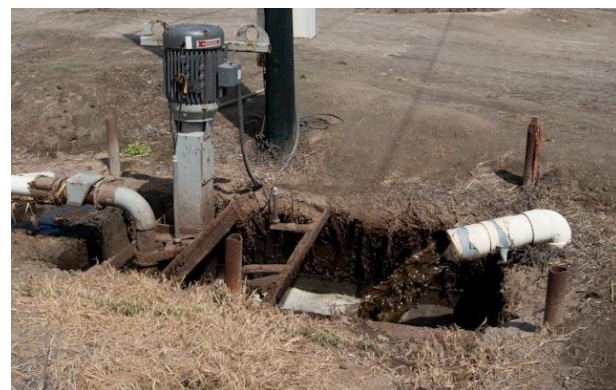
The flow rate of this liquid manure discharge could be estimated by timing how many seconds it takes to fill a 5 gallon bucket. If it takes 10 seconds, or 10 \div 5 = 2 seconds per gallon, then in 60 seconds (1 minute), 60 \div 2 = 30 gallons or 30 gpm would be pumped. Or, calculate gpm by dividing 300 by the number of seconds it takes to fill 5 gallons.
