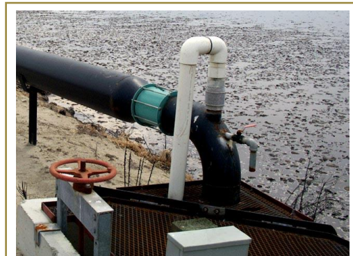
To calculate the amount of nutrients applied, a sample must be taken of the same material that is being measured. This sampling spigot is well-positioned for ease of use.
