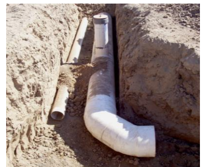
Two different pipe sizes were installed in the same trench to accommodate the range of application rates required by this operation.
