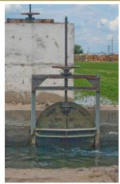
Slide gate valves such as this irrigation turnout are often used on gravity outlets of lagoons.
