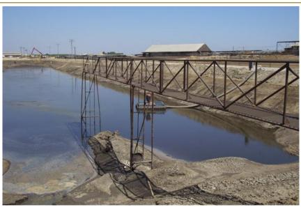
Valves in gravity systems are often accessed from a catwalk. If this valve is used for throttling, it will likely need frequent adjustments. Make certain that the valve can be accessed safely, especially in the dark. This pond has outlets at different depths in the pond, making it possible to adjust the amount of solids in the material being applied.
