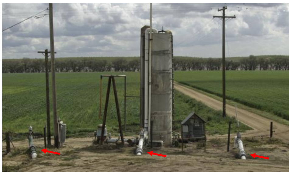
In this installation, separate metering runs allow lagoon water to be accurately applied on three locations simultaneously. A kiosk provides a lit, sheltered location to post target flow rates and record data.
