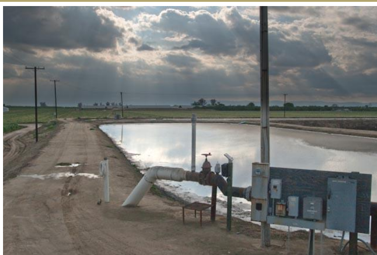
A flow meter on dairy lagoon discharge not only simplifies recordkeeping but enables the operator to accurately apply a predetermined rate of nutrients when used along with a flow control device such as a throttling valve.
