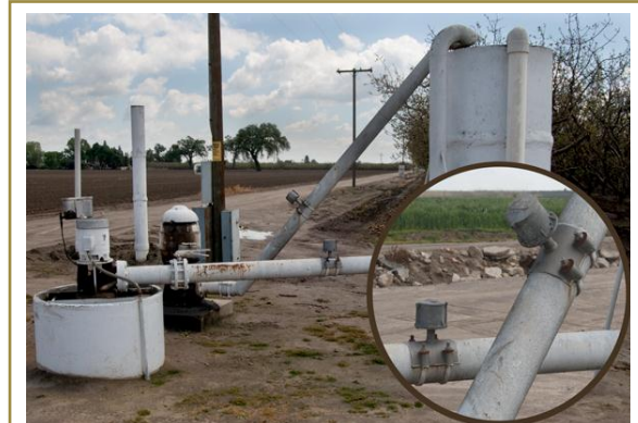
Inexpensive propeller meters are well suited for measuring pumped groundwater or clean district water but can easily foul if debris is present.
